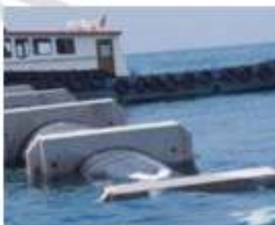
Marine Discharge Pipes
